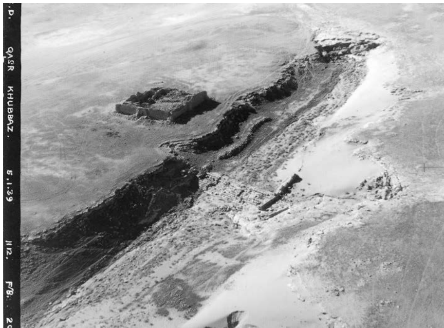
The castellum at Qasr Khubbaz. It was originally spotted and photographed from the air on 12 December 1938; the photograph illustrated here is one taken when Stein revisited in January 1939, which better shows the ravine and the remains of the barrage that was built across it to create a reservoir (ASA/3/261).
