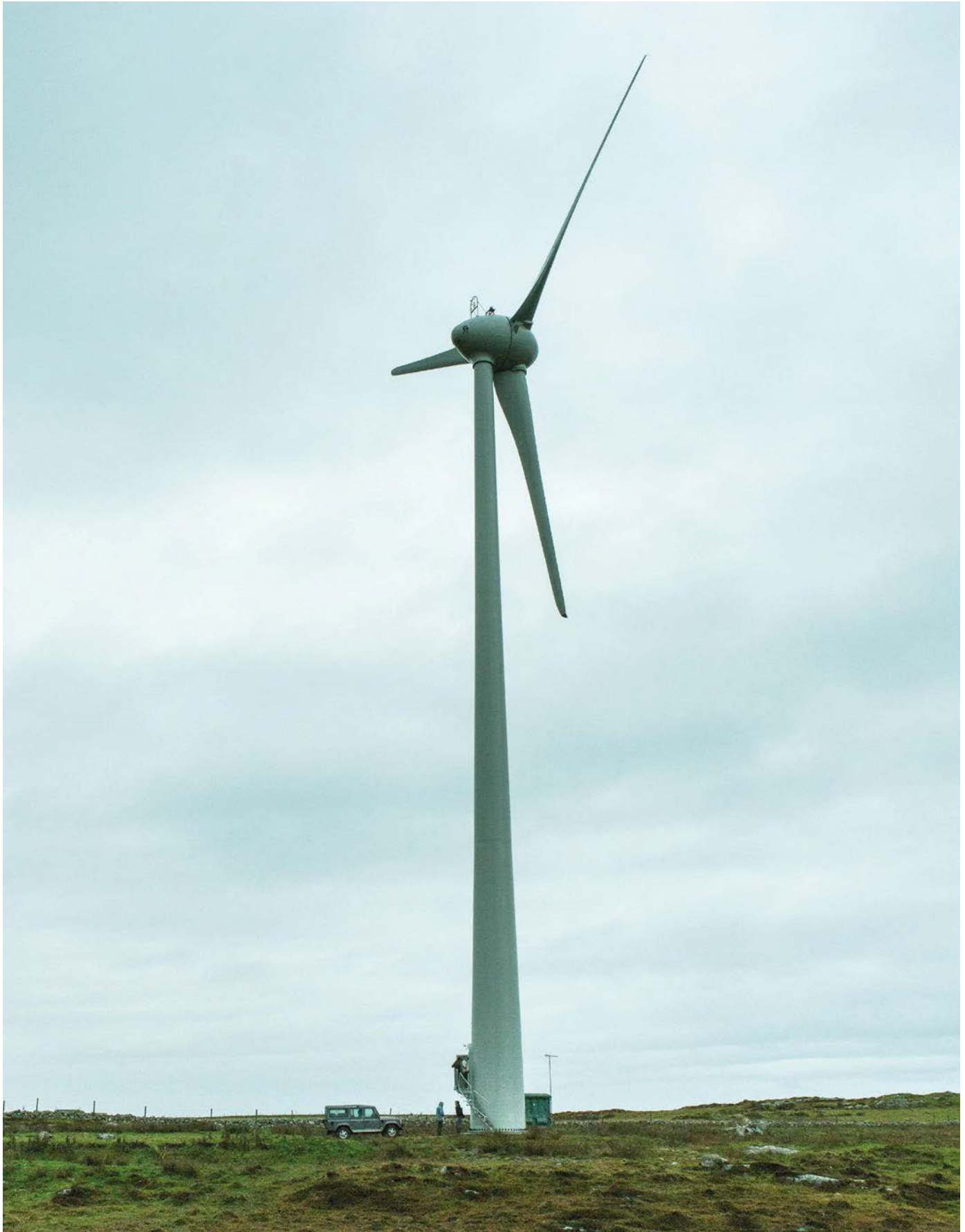
This wind turbine on Tiree generates electricity for the benefit of the community. Photo: Alamy
