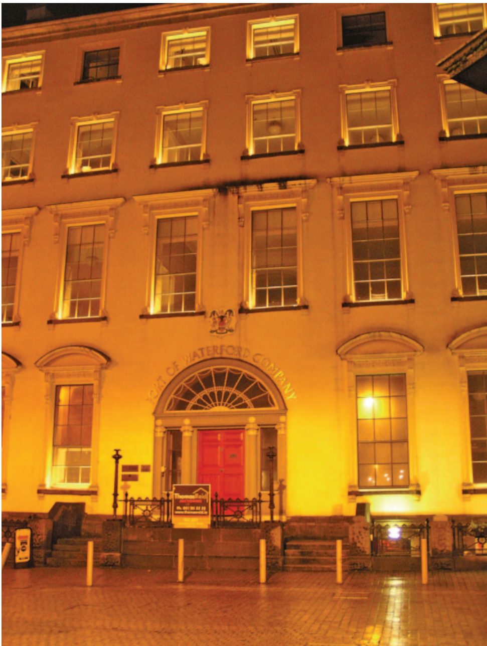
Figure 1. The Waterford chamber of commerce building, continuously occupied since 1815.
