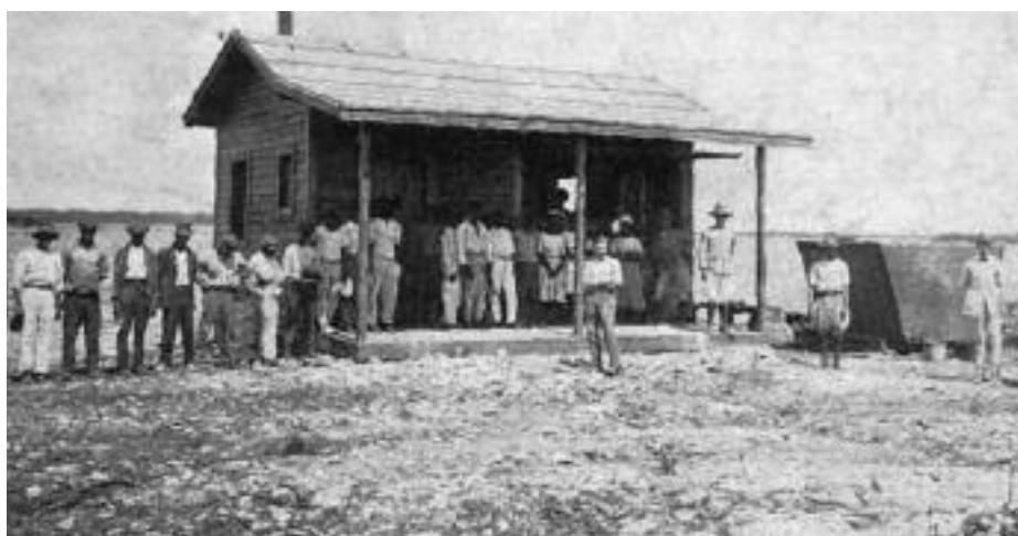
Kitchen at Cuban American Sugar Company's Quarantine Station, Puerto Padre, Cuba, 1920s. Photo from Agricultura y zootecnia.
